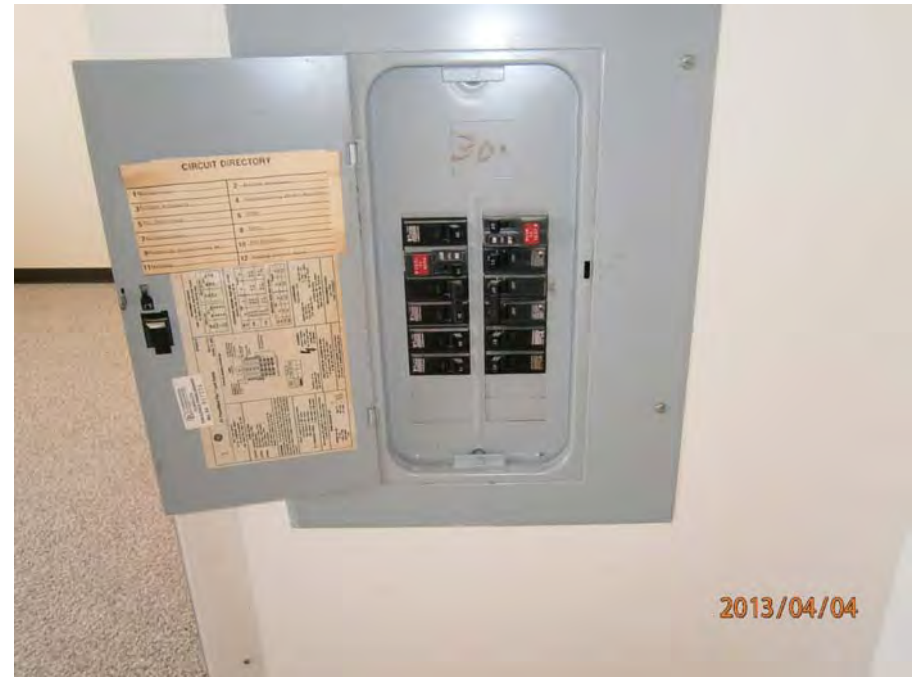
30. Unit circuit breaker panel
