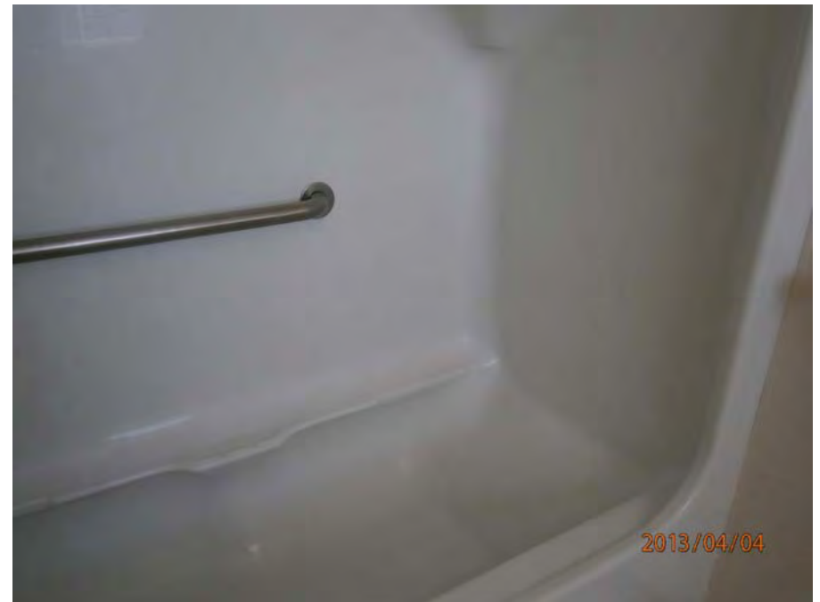
32. Unit tub seat missing
