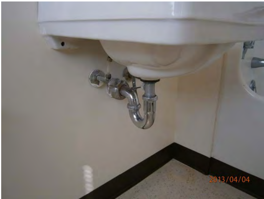
31. Unit sink trap protection missing
