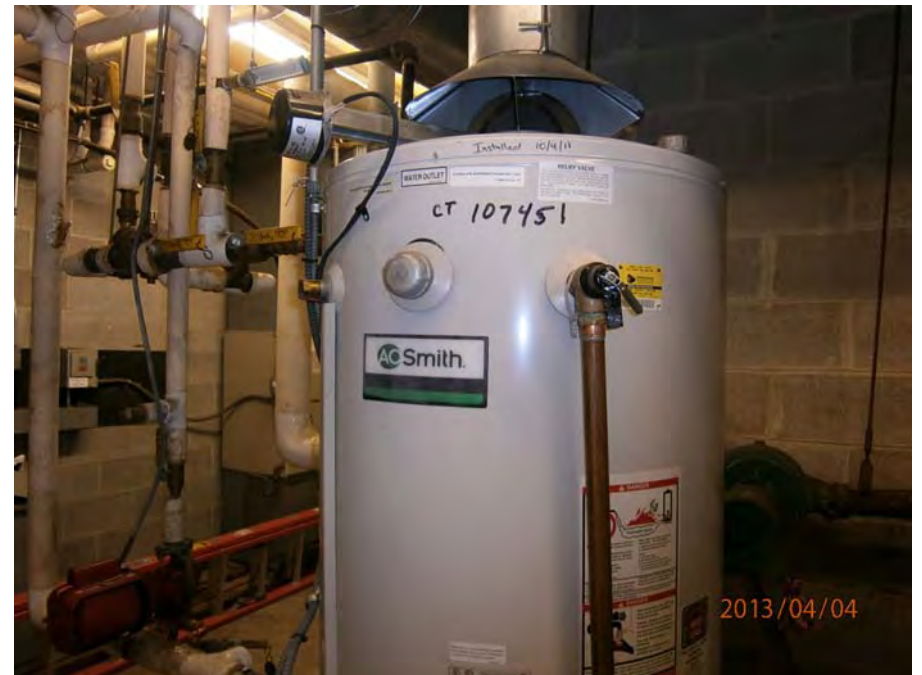
16. Gas-fired DHW tank
