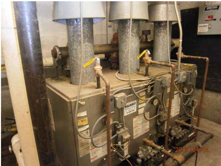
15. Gas-fired boiler
